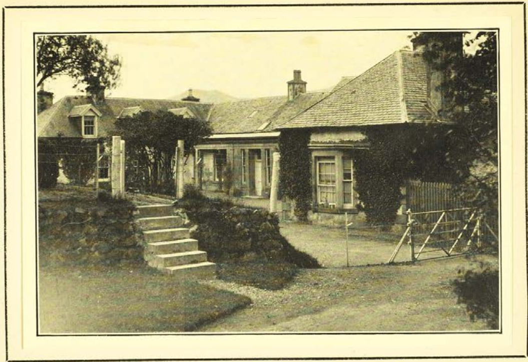
FRONT OF HOUSE AND COURTYARD
